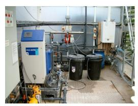
Water is recycled and run-off solutions are captured, filtered and recycled through the whole irrigation system. This enables a saving on water and nutrient use and avoids the pollution often associated with field grown crops.
