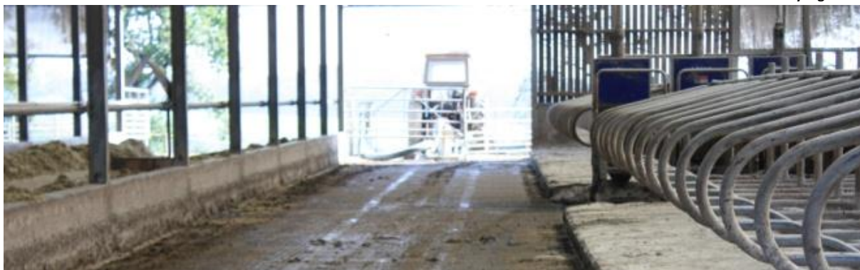
The slatted shed above the slurry lagoon
